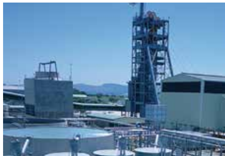
Designed and built water treatment plant to upgrade surplus fissure water to process, potable and service water quality
