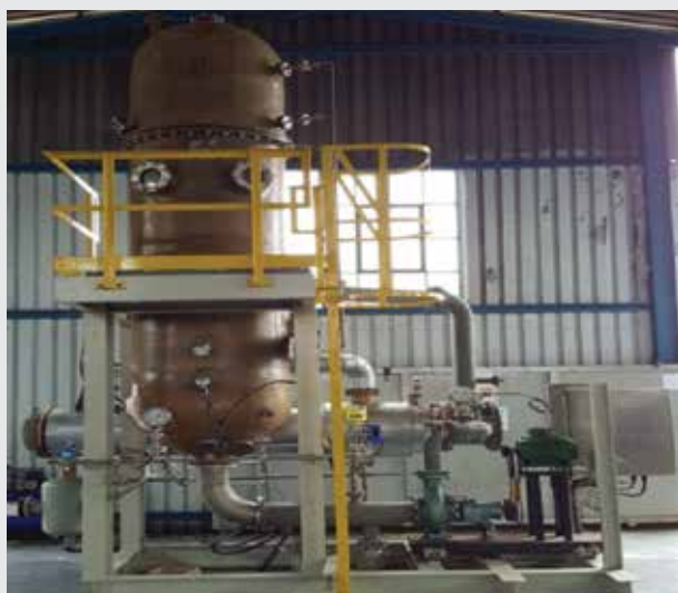
LP evaporator & crystalliser units. Using vacuum to reduce boiling points to reduce overall energy requirement for ZLD solutions of highly concentrated waste streams
