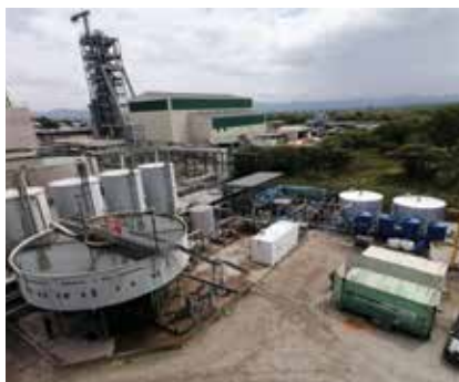
Designed and built water treatment plant to upgrade surplus fissure water and to process, potable and service water quality
